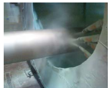
Shot Blasted Steel Pipe
